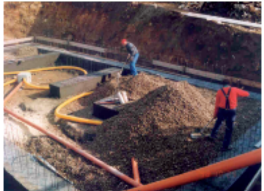
Incorporation of a radon drainage system in gravel
