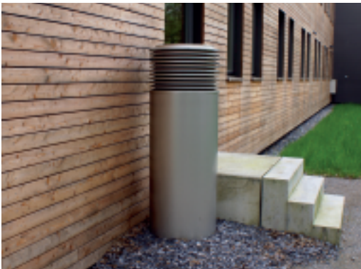
Inlet vent for controlled ventilation of inhabited rooms (at least 80 cm above ground level)
